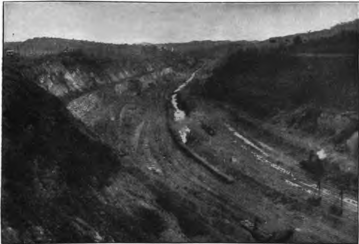
CULEBRA CUT LOOKING SOUTH FROM BEND IN EAST BANK NEAR GAMBOA.
